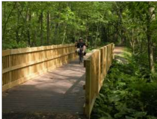
Trail and bridge example in nearby Clifton Park.
