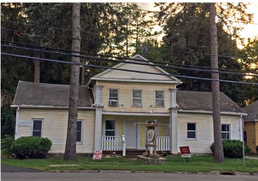
Former Boarding School 1854
